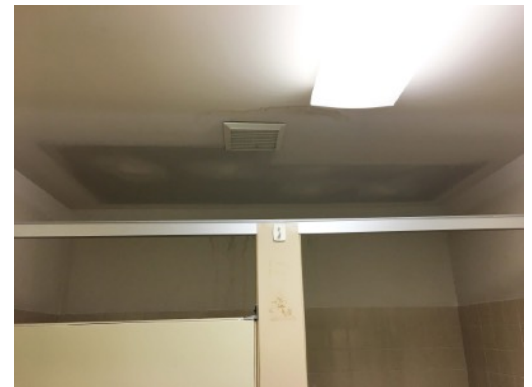
The drywall water damage was repaired, then our members went to work finishing it.
